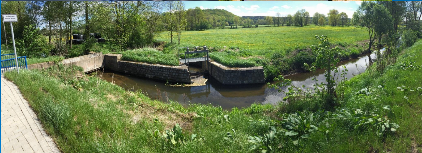
The first kilometers - The dam and the old raftsmen house in Crossen (Thuringia) and technical facilities near Pötewitz (Saxony-Anhalt)
